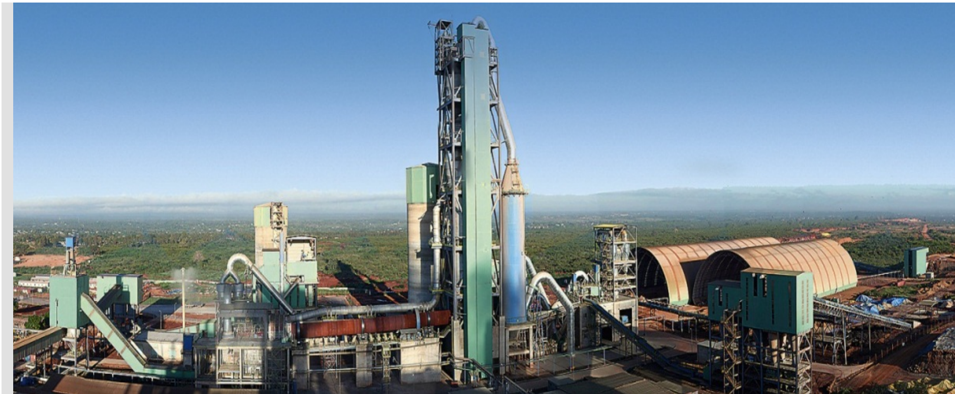
Tanzania Portland Cement, Werk Wazo Hill, Tansania
