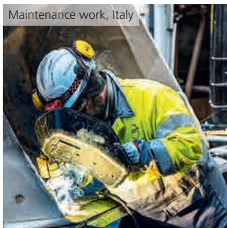
Maintenance work, Italy
