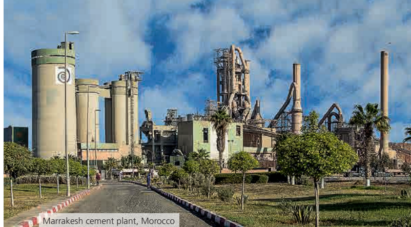
Marrakesh cement plant, Morocco
