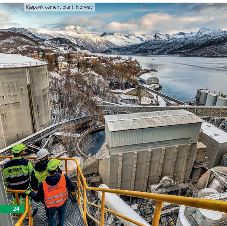
Kjøpsvik cement plant, Norway
